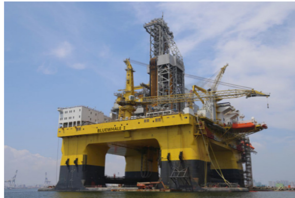
世界钻井深度最大的半潜式钻井平台“蓝鲸1号” The world-wide deepest semi-submerged drilling platform “blue-whale 1#”
